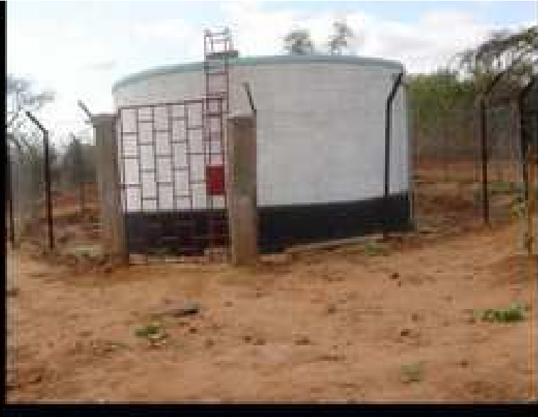
Wambiti distribution water tank (100m 3 ). The tanks are fenced for sanitation purposes.
