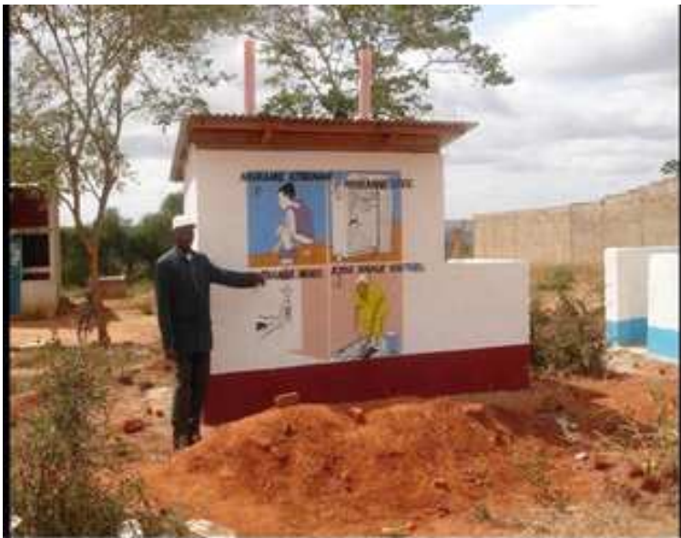
A public sanitation facility with murals depicting common sanitation and hygiene practices in the development areas. Murals such as the ones in the photograph have proved to be very effective in behavioural change.
