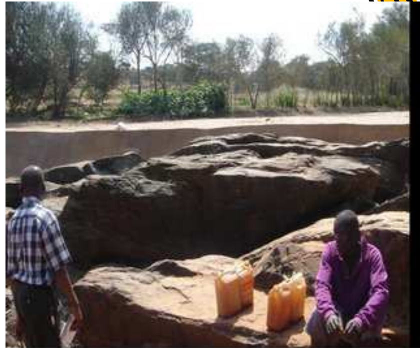
Muhi sub surface dam. Water is stored underneath the sand.
