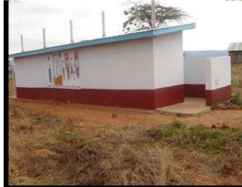
The situation has been improved in Wambiti Primary School by the construction of improved VIP latrines in the school. Murals have been drawn for behaviour change purposes. No more waiting hence time saved for academic purposes.
